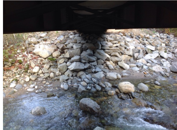
Right Bank Abutment when facing downstream
