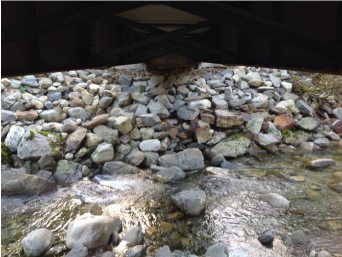
Left Bank Abutment when facing downstream
